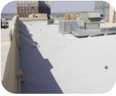
application as well as improved long-term performance. SA-APP Cap Sheet is also used as a flashing membrane in all applicable specifications. Meets ASTM D6222 Type 1, Grade G (granular) / ASTM D1970.
