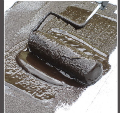
Mule-Hide #301 Fibrated Emulsion Roof Coating being applied with a roller.
