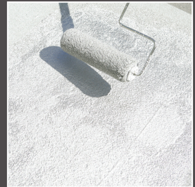
Mule-Hide #401 Premium Fibrated Aluminum Roof Coating being applied with a roller.
