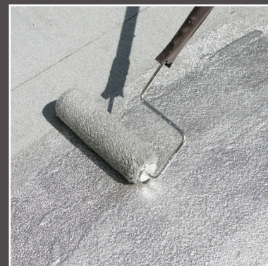
Mule-Hide #416 Standard Non-Fibrated Aluminum Roof Coating being applied with a roller.
