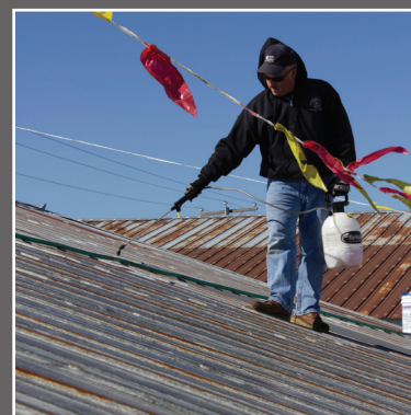
Using airless sprayer.
