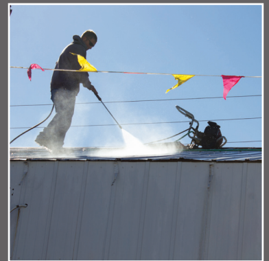
Power washing metal roof.
