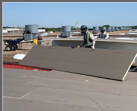
Application of 4'x12' panels on the roof deck.
