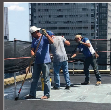
Application with 3/8" nap roller
