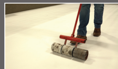
Using 75 lb. roller to secure attachment to substrate.
