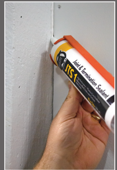
Sealing a joint with white JTS 1 joint and termination sealer.
