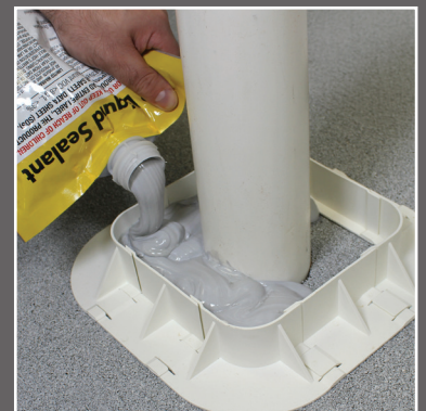
Applying to a pitch pan.
