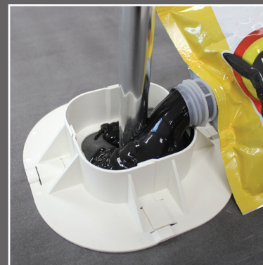
Horizontal installation with MP Liquid Sealant
