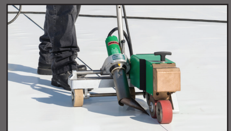
Heat Weldable Seams
