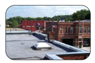
Fire Retardant (FR) EPDM membranes are specially formulated to inhibit spread of flame and meet or exceed code body testing criteria for fire retardant roofing membranes.
