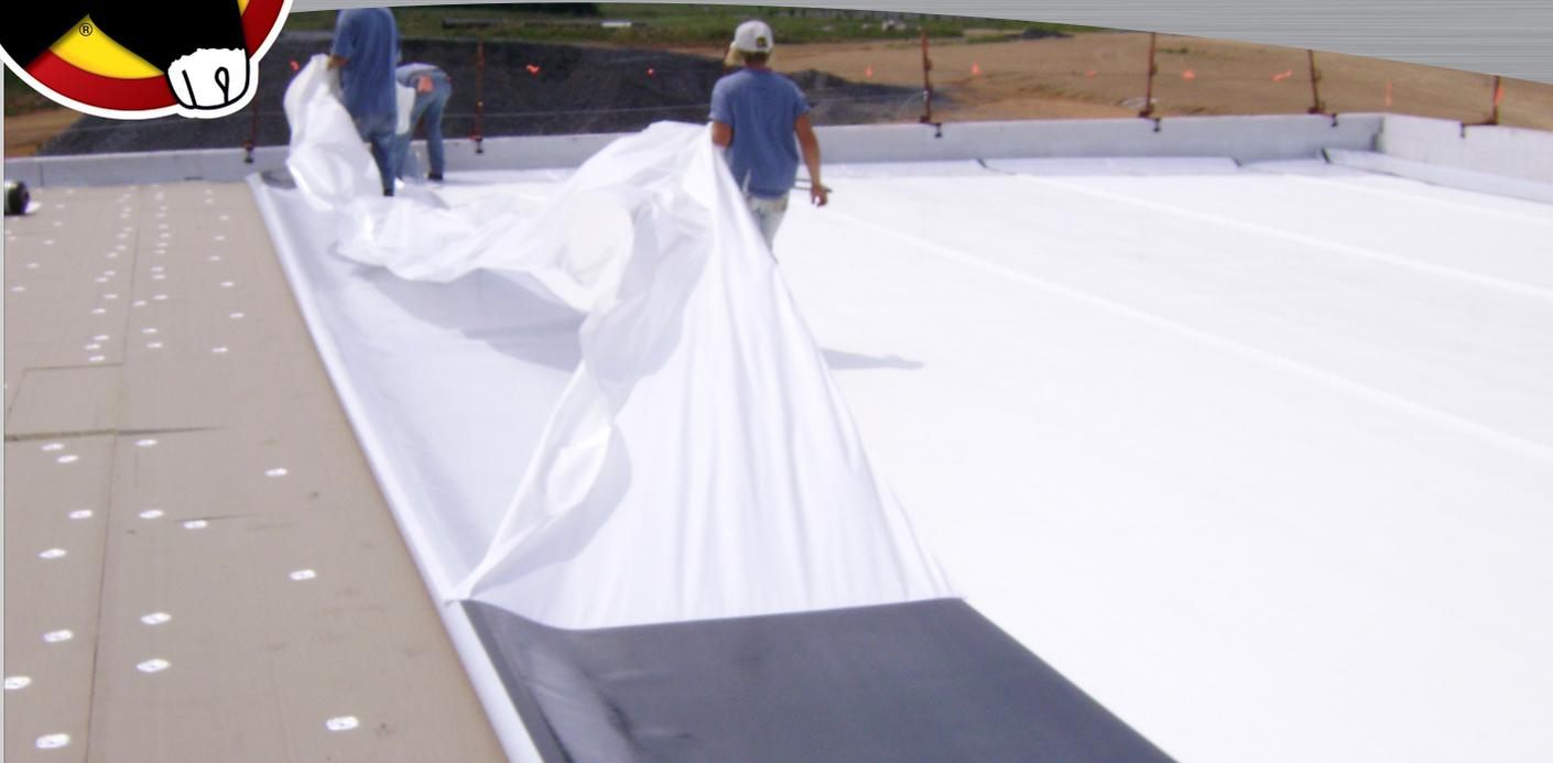
SA-TPO is a 60 mil white TPO membrane laminated to a pressure-sensitive adhesive. It is packaged in 10' x 50' or 10' x 100' rolls. There is no lead time on this product, and it can be top loaded with other TPO or EPDM orders shipped from Carlisle, Penn., Senatobia, Miss., and Tooele, Utah.
